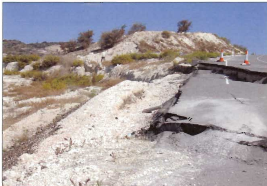
Fig. 6: Landslide at Pentalia - Statos road.
